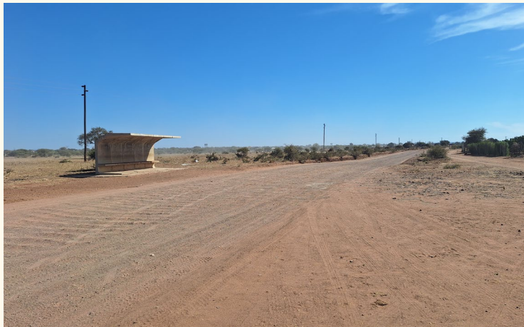
Throughout the villages, work has been done to provide bus shelters.
